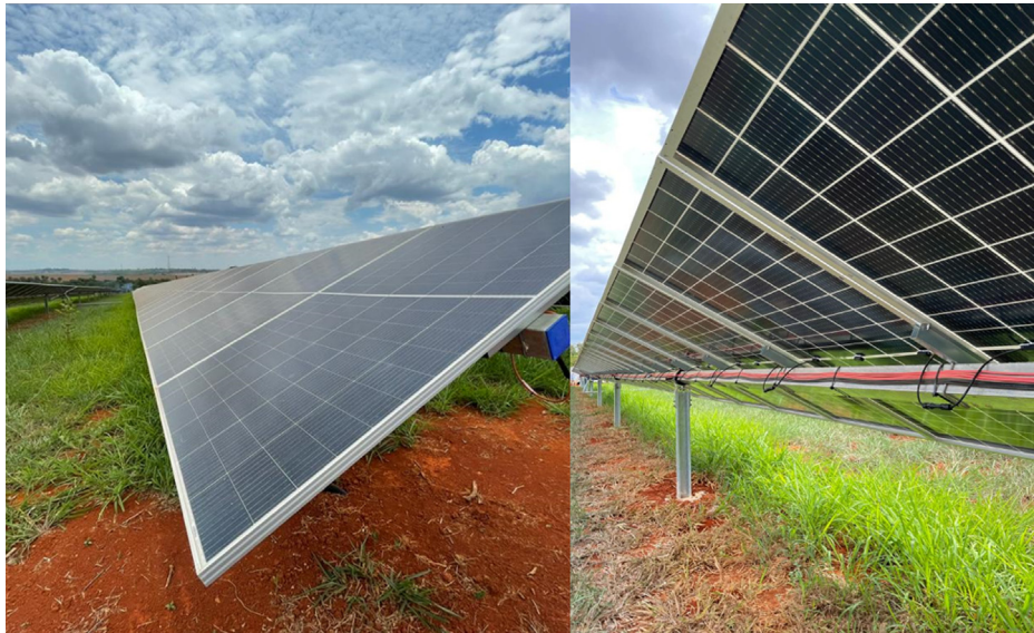
Fig. 9. Details of the ground conditions at the Iguatama Solar Power Plant.
