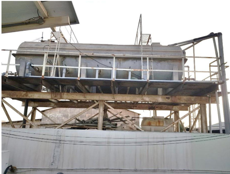
Fig. 2. A large desalination tank (silo) – located at azimuth from nearly 240° to 280° (west-south to west) and higher than the roof level by nearly 10 m causes shading effect to the PV rooftop system on House #3 which led to less solar electricity yield.
