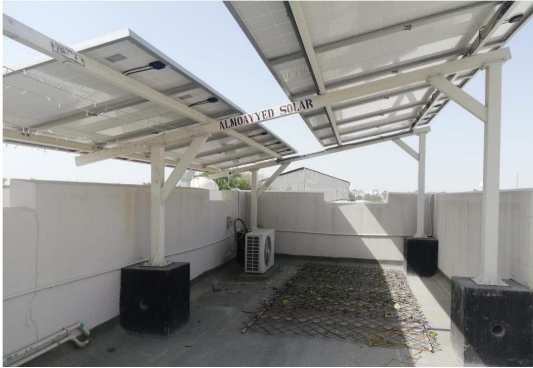
Fig. 1. The PV panels on the rooftop of the first 7.8kW – PV domestic building (House 4 #108) in Bahrain were anchored on Concrete Foundation that can withstand wind speed no more than 30 m/s (110 km/h).
