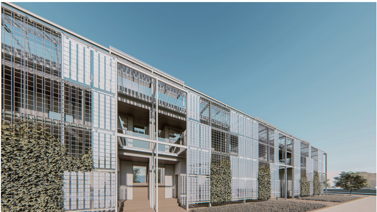
Fig. 6. Active exoskeleton with photovoltaic glass panels and green shielding on building B.
