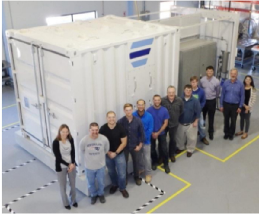
Fig. 7. Image of a module of “Ambri” Liquid Metal battery bank, part of the contract with NEC 200 MWh project [9].
