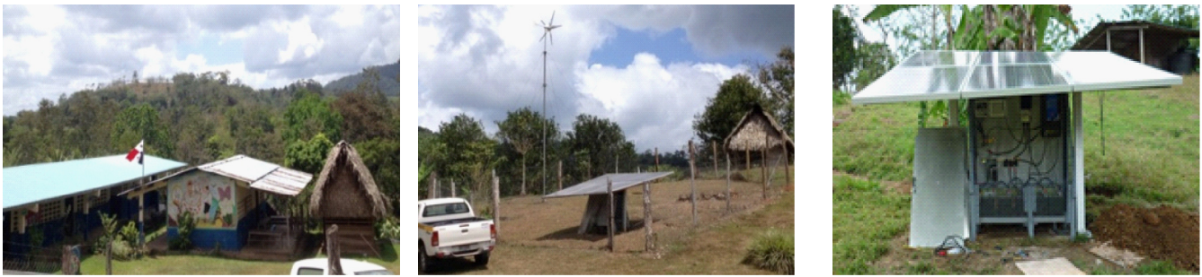
Fig. 1. Boca de Lura school facilities and power plant views.
